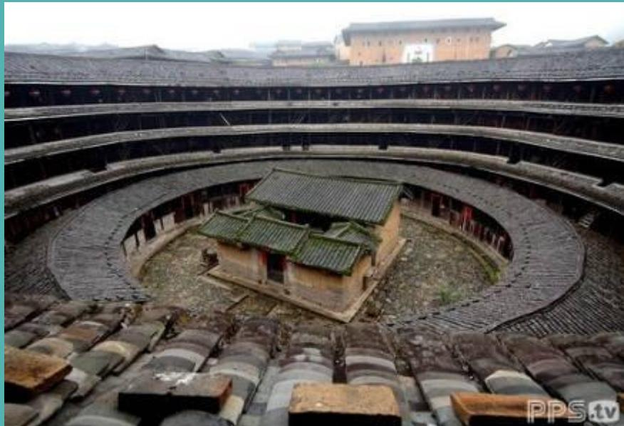
The end result is a well lighted, well-ventilated, windproof and earthquake-proof building that is warm in winter and cool in summer. Tulous usually have only one main gate, guarded by 4-5 inch thick wooden doors reinforced with an outer shell of iron plate. The top level of these earth buildings has gun holes for defensive purposes.
