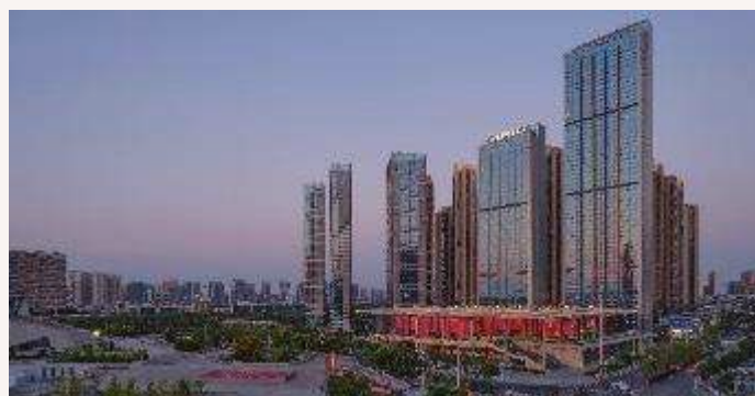
长沙北辰会议中心 Changsha North Star Convention Center 建筑面积4万平米 40,000 square meters building area
